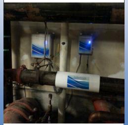
Mark-III installed on 6" pipe.
